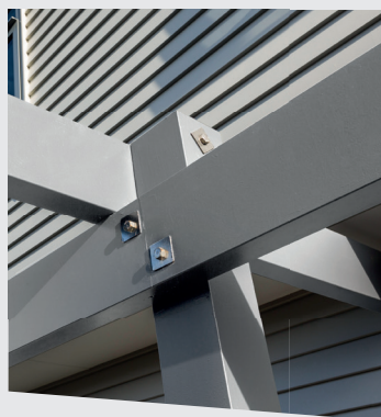
POSTS, BEAMS & CLADDING
