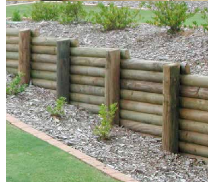
A unique look. Koppers Roundback sleepers, profiled from 175mm half rounds look great and are a more durable alternative to standard landscape pine sleepers.
