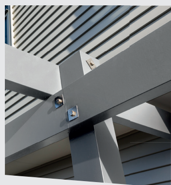
POSTS, BEAMS & CLADDING
